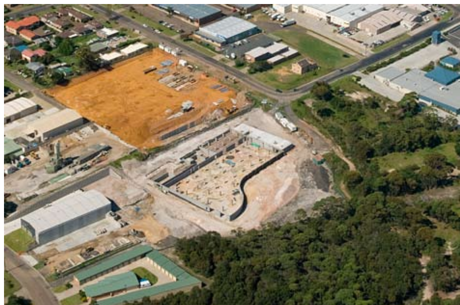
Site progress February 2008
